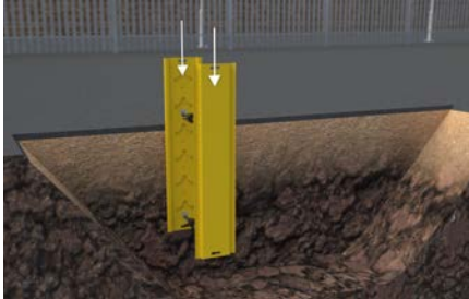
Figure 10 Lift the EZE Hub pile sub assembly and position at the top of the battered end of the excavation – 2 persons required. With one person either side of the excavation, lower the sub assembly into position.
